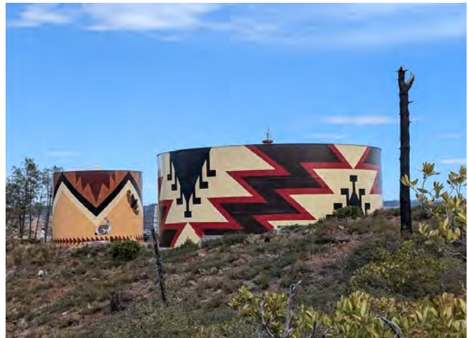
The painted tanks seen from a distance.
